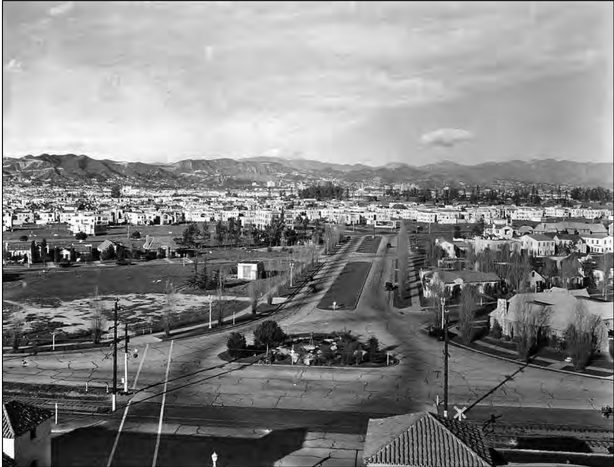
Figure 10. View to north up S. McCarthy Vista from the roof of the Carthay Circle Theater, ca. 1930. Source: waterandpower.org.
